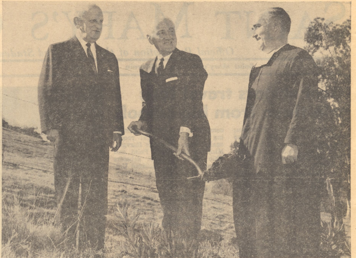
Ground for two new dormitories at Saint Mary's College is ceremoniously broken by Daniel J. Cullen, president of the board of regents, while another regent, Fred A. Ferroggiaro of Oakland, and president of the college Brother Michael Quinn, FSC,
