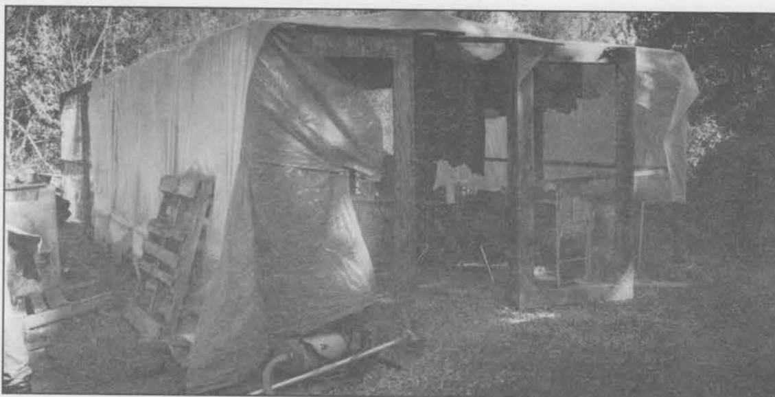
Maintenance workers eat lunch in this structure behind Assumption Hall.
