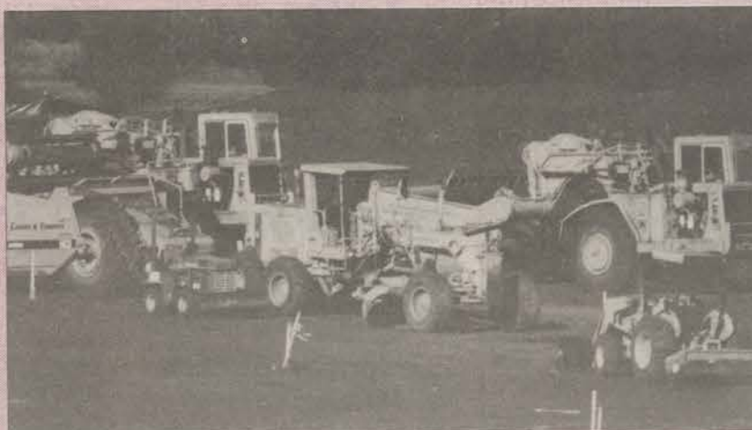
Construction sight of future Softball Field.
