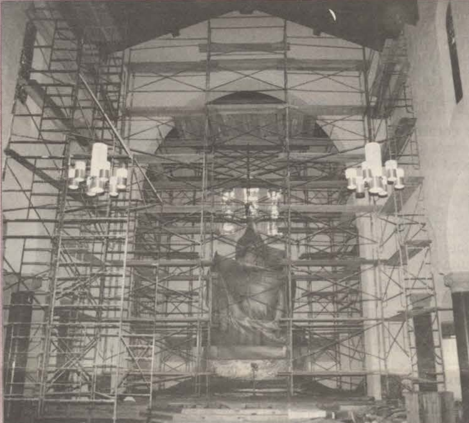
The Chapel under Phase III renovation.
