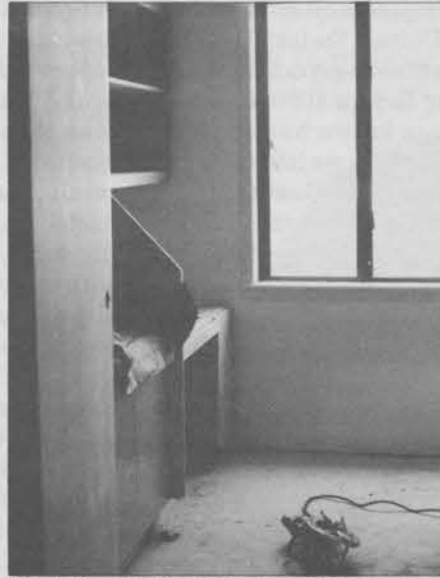
Augustine dorm under construction.
