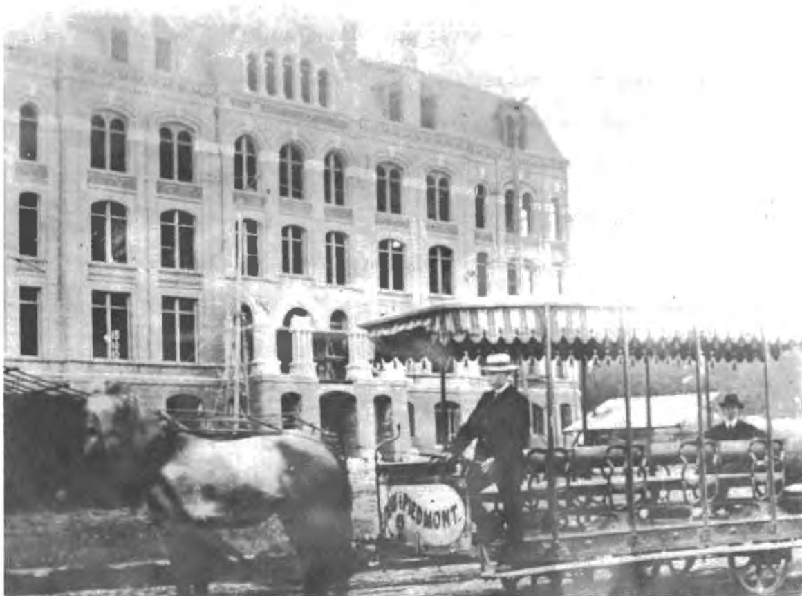
St. Mary's College Under Construction, 1888
