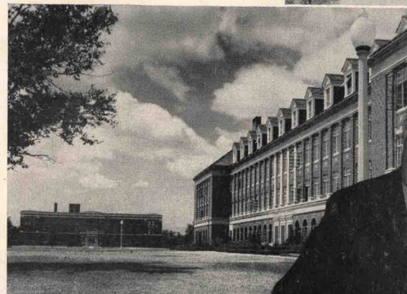
Below - Whitehurst Hall (Administration Building) with Infirmary in background
